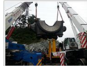
Seating the Exist LP Lower Casing
