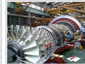
Blade Ring Assembly & Bolt Tightening
